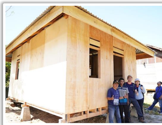
Transitional Shelter at Central Sulawesi
