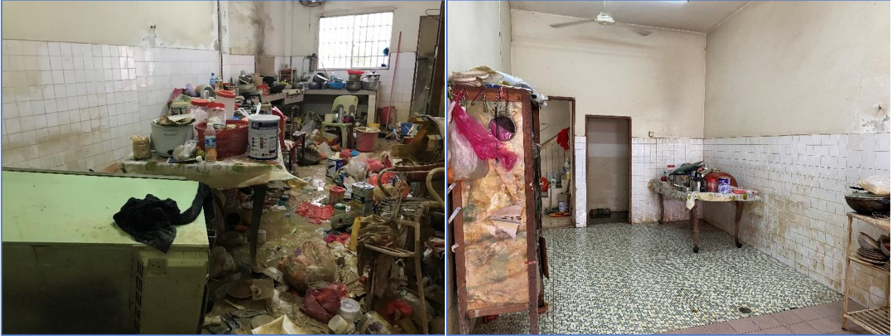
The before-and-after photos of the house of a single 83-year-old Chinese lady staying alone. As she collects recycled items for a living, the photo on the left showed the devastation of her house caused by the flood.
